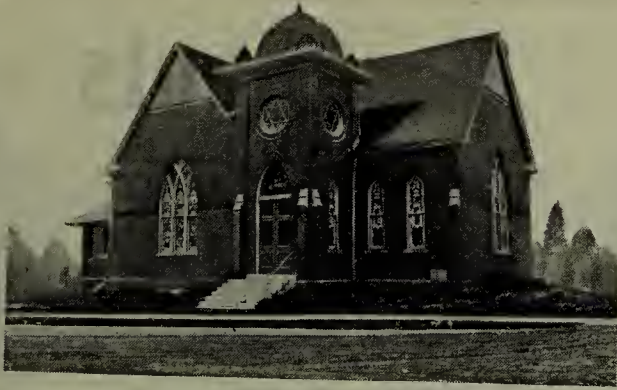
Church at Albany, Missouri, heated with a battery of two No. 490 Gilt Edge Furnaces.
